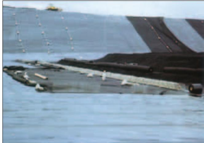
The short-term load effect from building up the drainage gravel can be simulated by construction tests on site. Such field trials using construction machinery and materials supplied by the contractor provide the opportunity to check the design of the protective system and minimise the impact on the geomembrane.
