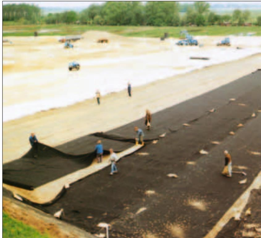
The standard protection requires a needlepunched nonwoven with a unit mass of at least 1200 g/m<sup>2</sup> and a 15 cm thick layer of crushed aggregate (0 - 8 mm) on top of the geomembrane. These two layers provide sufficient protective efficiency. When placing an aggregate drainage layer (16 - 32 mm), HaTe® reinforced nonwovens or other composites are often used to replace this standard protection, when specific site conditions are difficult for the installation.
